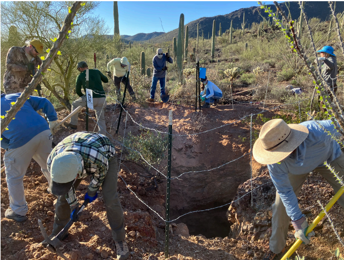
Volunteers working to fill a 12-foot deep mine shaft in Tucson Mountain Park.
